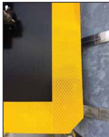
Exhibit 8: Installation details for retroreflective borders on backplates. The photo to the left shows where the backplate was cut along the bottom to fit around the signal head. The backplate was fastened to the signal housing to the left and right of the cut. The photo to the right shows a detail of the applied tape. (Source: VHB)
