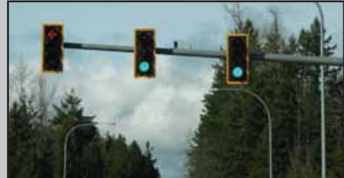
Exhibit 11: Mast-mounted signals with retroreflective borders. (Source: VHB)
