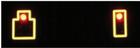
Exhibit 2: In June 2005, yellow retroreflective borders were added to existing backplates at three high-crash locations in Columbia, South Carolina. Simple before- and after-implementation comparisons showed crash reductions at the three sites ranged between 29 percent (total crashes) and 50 percent (late-night/early-morning crashes). 5 (Source: FHWA)
