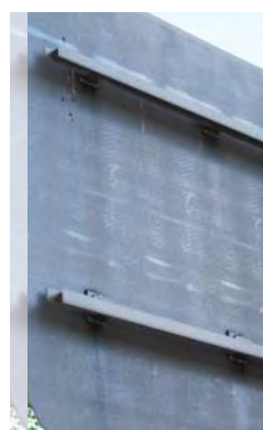
Aluminum Z-bar on an overhead guide sign
