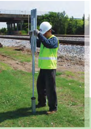
Anchor installation with a Universal Slide Hammer
