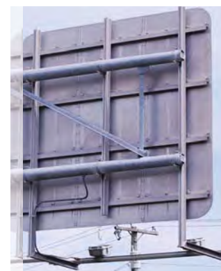
Aluminum Z-bar on an overhead guide sign
