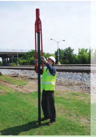
U-Channel post installation using a manual post driver
